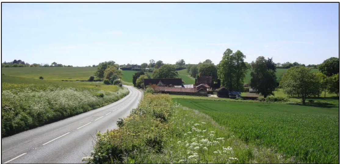
Fig.45 View WSW from Hadleigh Road East (VP3)
